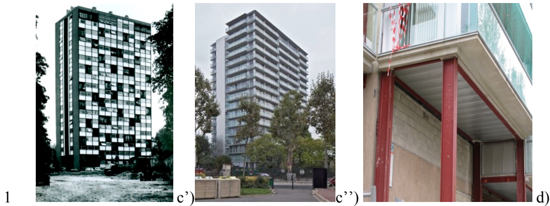
1 2 Figure 1. Non-integrated approach: a) post-earthquake scenario of energy saving measures carried out 3 disregarding structural vulnerabilities (retrieved from: ADNKronos); b) structural retrofit carried out 4 disregarding architectural context (www.studiomapi.it). Example of partially integrated approaches: c') 5 and c'') ante and post camouflage intervention of Tour Bois-Le-Prêtre, Paris by Druot, Lacaton & 6 Vassal, 2012; d) detail of the self-supporting exoskeleton, independent of the existing structure (Angi 7 2016).
