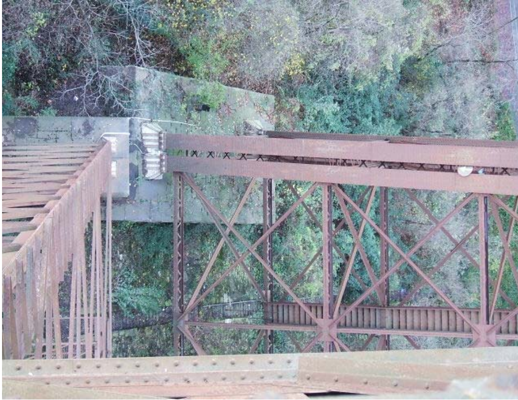
Fig. B5: Particular of the shoulder of the arch and the big pier on the Paderno bank.
