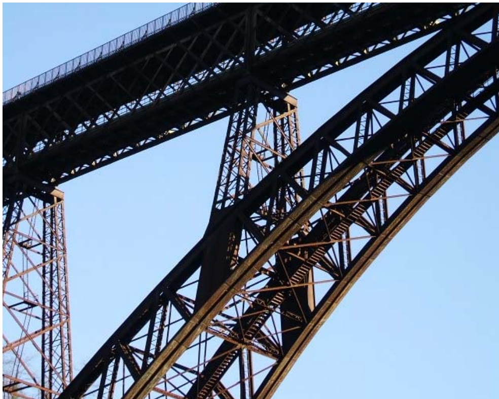
Fig. B2: Bottom view of the arch/pier/upper beam connection.
