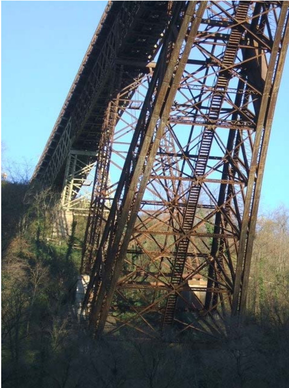
Fig. B4: View of the shoulder of the arch and the pier on the Calusco bank.
