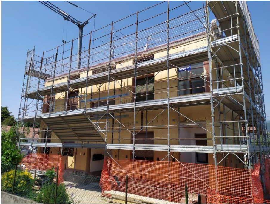
Figure 2. Case study 2: CLT exoskeleton with coupled shear walls (Zanni 2023)
