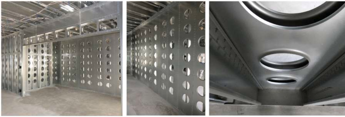
Fig. 1. Examples of real applications of steel sheet shear walls with burring holes.
