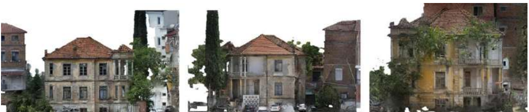
Figure 8: Villa's photogrammetric facades
