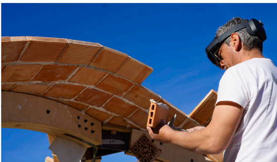
Fig. 3. Augmented thin-tile vault construction using digital guidework.
