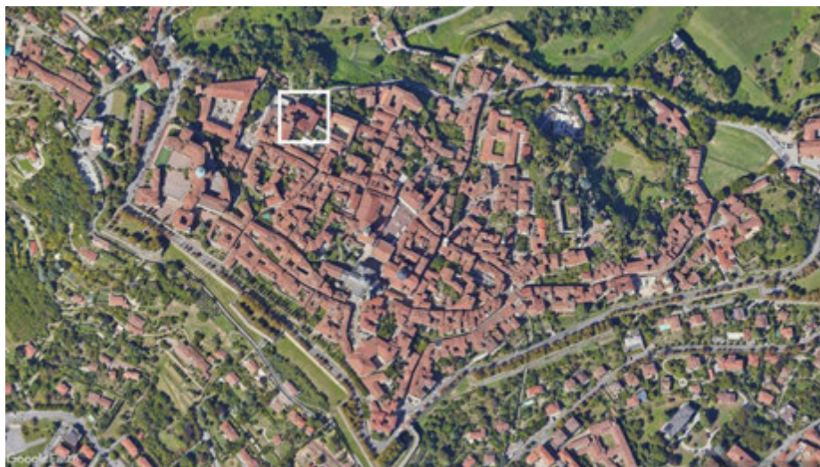
Fig. 2. The image identifies the former Carmine Monastery complex (white rectangle) within the historic city (source: Google Earth)
