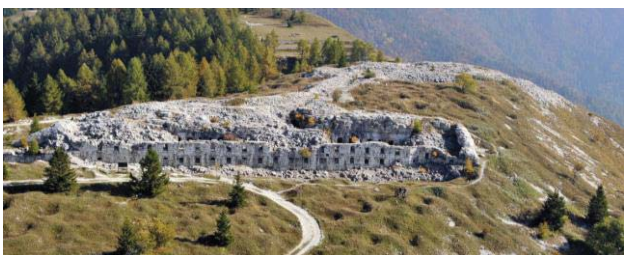
Fig. 3 - Surroundings Serrada Fort
