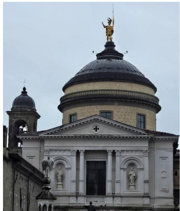
Fig. 1. Exterior view of the dome of S. Alessandro.
