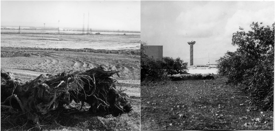
Figure 3. Excavation July 1961 (left) and Excavation December 1961 (right). Source: Archivio di Stato di Taranto (1961a, 1961b).
