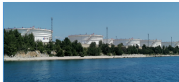
Img. 3: Five of the twenty oil tanks owned by Janaf, the Croatian national oil company ( Photo by the author ).
