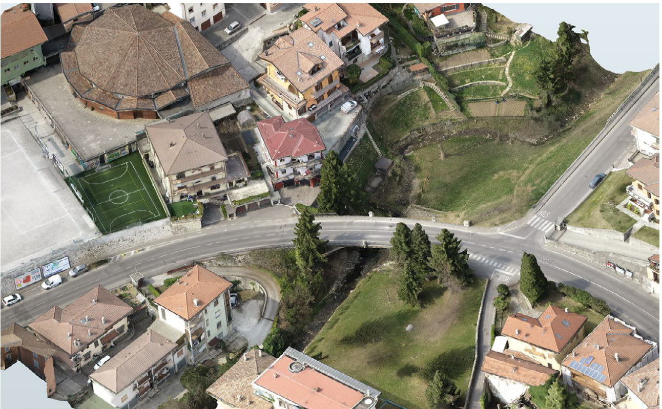
Figure 5: Nembro bridge: 3D model. Photogrammetric and TLS-based reconstruction of the bridge geometry. Image credit: Cardaci, Versaci, Azzola (2023) [50].
