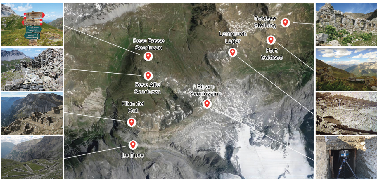
Figure 1: Stelvio Pass: overview of high-altitude military works. Composite view with a satellite basemap highlighting the principal First World War installations in the Ortles–Cevedale sector, including Filon dei Mot , Le Buse , Rese Alte Scorluzzo , Rese Basse Scorluzzo , Riparo Scorluzzino , Fort Goldsee , Goldsee Stellung , and Lempruch Lager . The lateral photographic strips provide on-site views and documentary frames that contextualise the remains and illustrate their current state of preservation. The figure establishes the spatial framework adopted in the chapter and locates the Filon dei Mot survey within its territorial setting and historical landscape. Image credit: [42].
