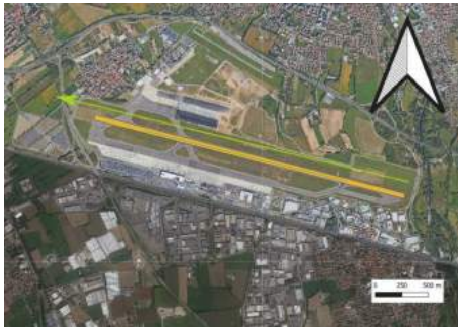
Fig. 13. BGY airport runway (yellow) with take-off/touch-down line (blue).
