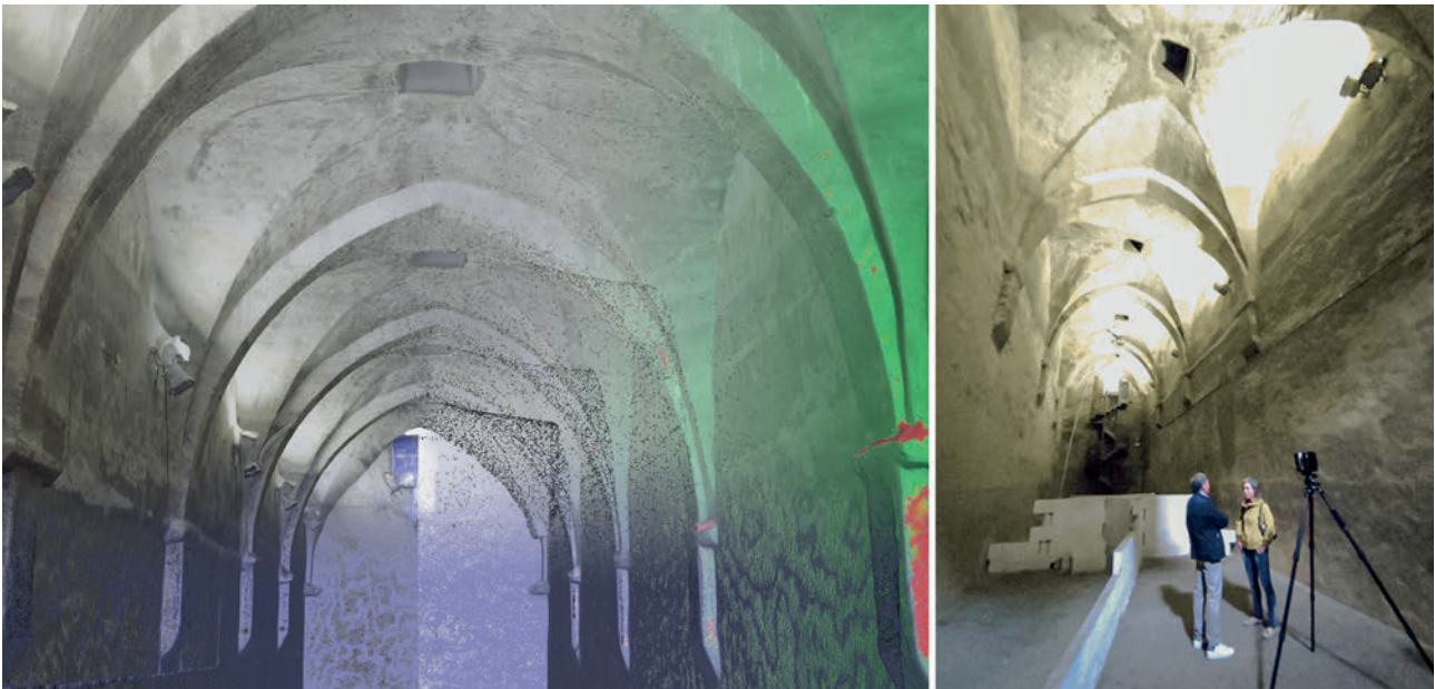
Figure 2. Internal area of Fontanone Visconteo : 3D photogrammetric models mix (overlap between point cloud, mesh texture and confidence indication).
