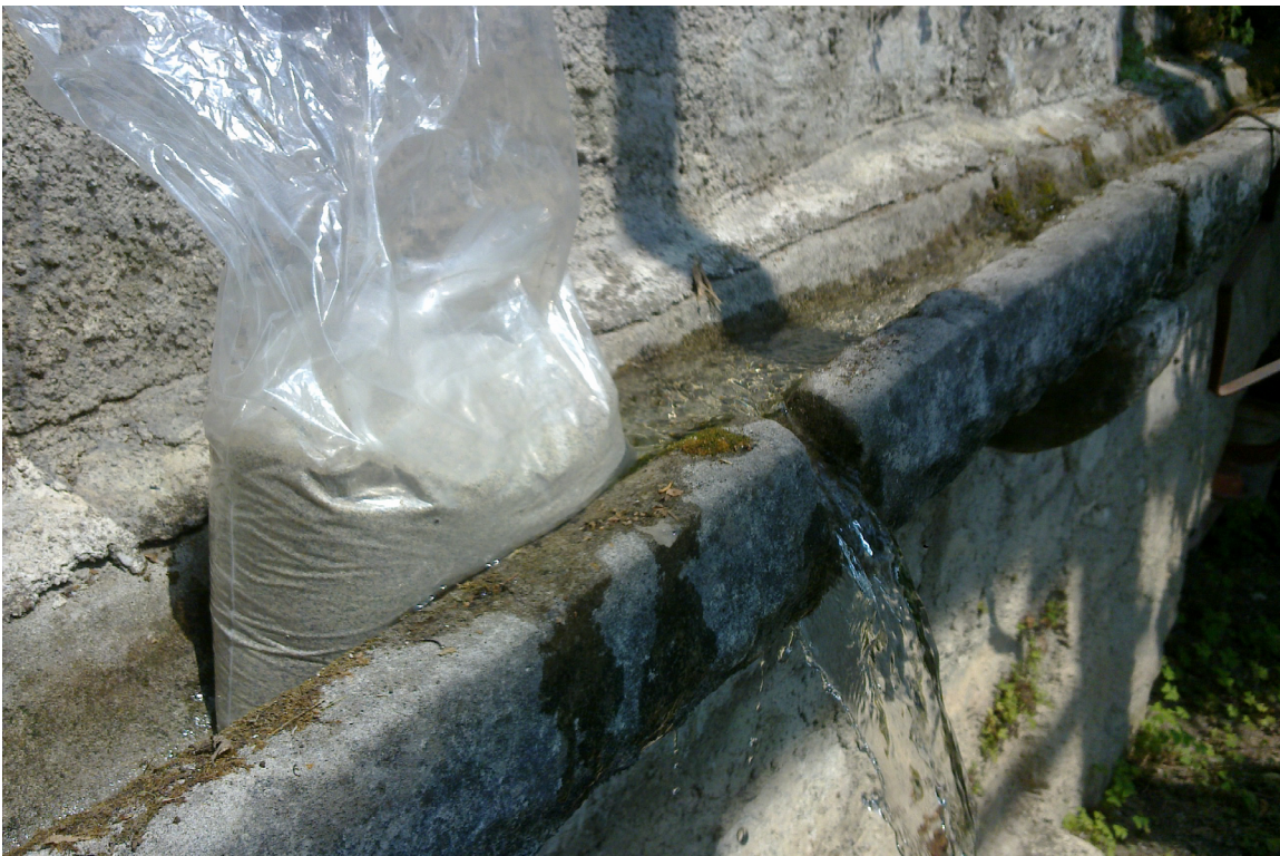
Figure 4: Activated spillway during an irrigation test at Limonaia La Malora (Gargnano; Brescia Province).
