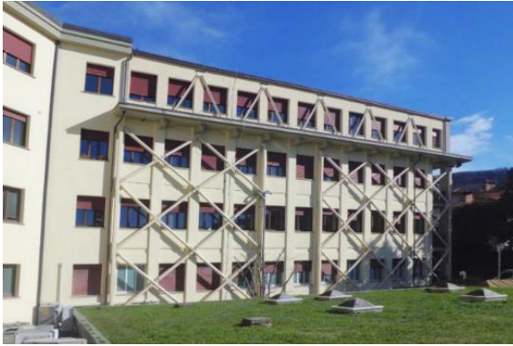
Figure IV.6 - External steel bracing for seismic retrofitting of a hospital building. From [82]
