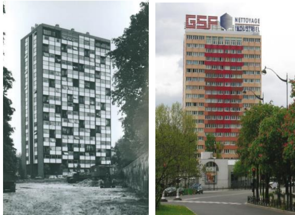
Figure IV.29 - On the left side: photo of the main façade at the end of construction, taken by the designer Raymond Lopez in 1959. On the right side: photo of the same façade after the first energy-efficient renovation, taken in 1990. From [135].
