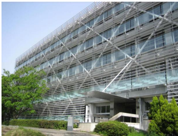
Figure IV.33 - Midorigaoka 1 st Building, Tokyo Institute of Technology: retrofitted building façade. From [137].
