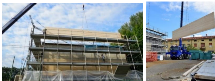
Figure VIII.39 - Pictures of the prefabricated structural retrofit under erection. From [15].
