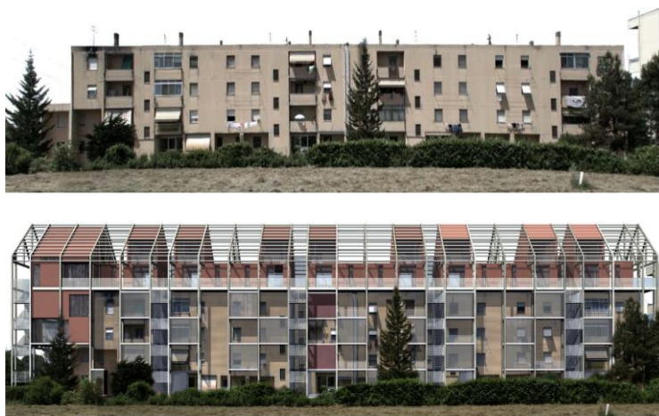
Figure IV.31 - On the top: main façade of the pre-existing buildings before renovation. In the bottom: the same facade after the intervention. From [136].
