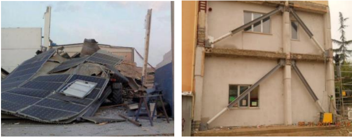
Figure II.2 - Traditional uncoupled refurbishment approach: the collapse of the solely-energy retrofit of an industrial warehouse renovated with photovoltaic panels after the Emilia-Romagna earthquake (2012) (left); solely structural retrofit: a typical seismic retrofit of an existent building through dissipative bracings (right). From [9].
