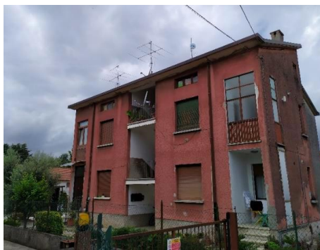
Figure IX.1 - View of the main façade before the intervention. Form [247]
