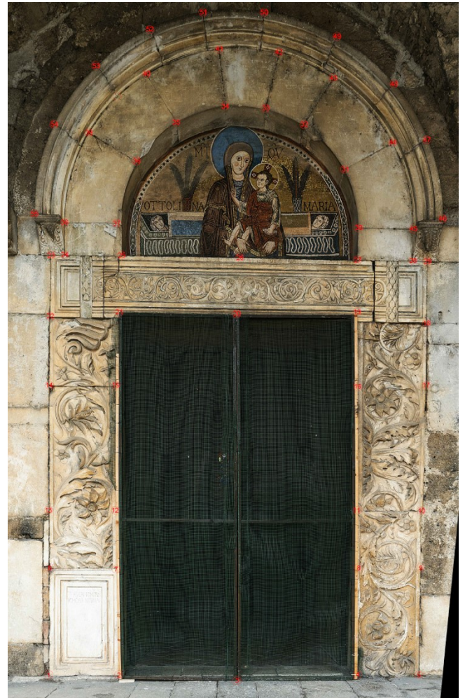
Figure 10. Main portal of the Church of Santa Maria della Libera: rectified orthophoto-plan obtained using DXO software, showing control points subject to direct survey.
