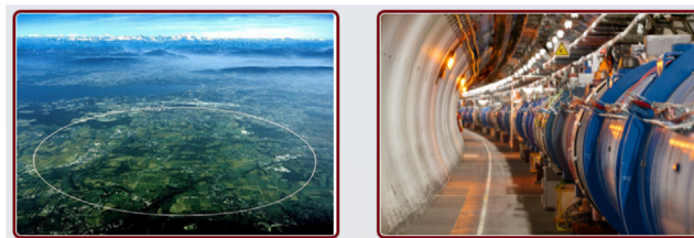
FIGURE 1 | The 27-km LHC tunnel, housing the LHC accelerator, here showing the superconducting magnets containing the two beam pipes [27].
