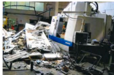
Fig. 13. Observed damage patterns following the 29 May 2012 earthquake: collapse of roof elements (left) and consequent damage to building contents (right).
