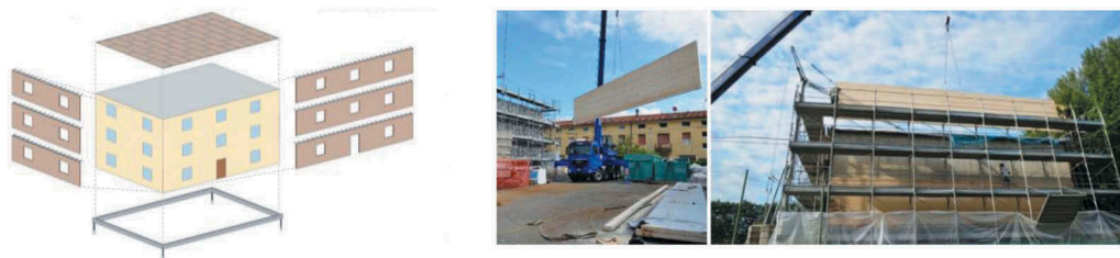
Figure 3. An example of LCT-based integrated retrofit intervention (from Zanni et al. 2021).
