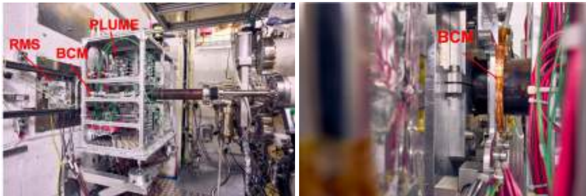
Figure 5. Left: RMS (under the mylar protection foil at the left side) and PLUME (inside the scaffolding). The arrow indicates the position of BCM which is hidden behind the PLUME scaffolding. Right: upstream BCM detectors inside their kapton-insulated support surrounding the beam pipe.
