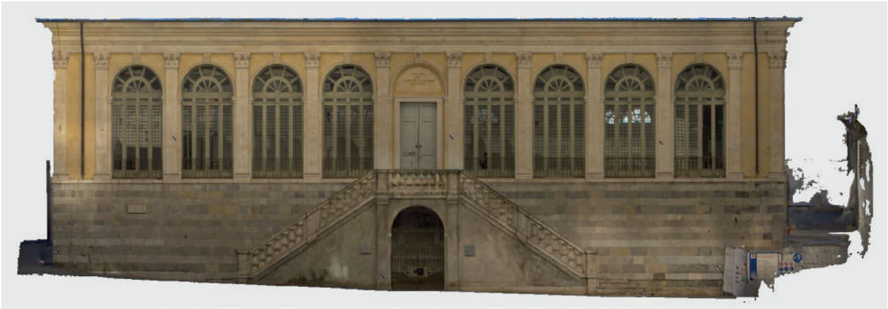
Figure 10. The Palazzo dell'Ateneo and the Fontanone : orthographic projection of the facade (© Lab_S.A.B.E.).
