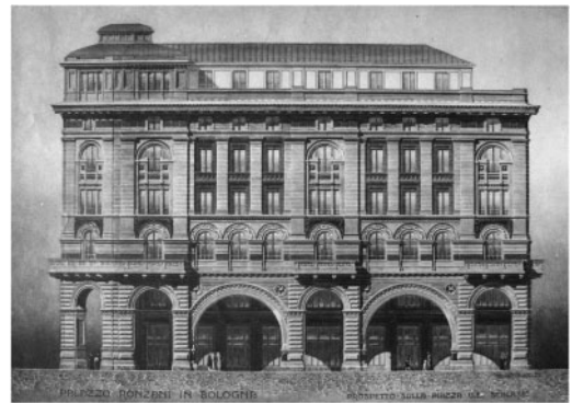
Figure 3. Main facade of Palazzo Ronzani (private collection).
