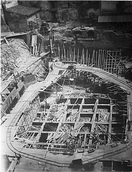
Figure 4. Construction phases of the foundation slab (private collection).
