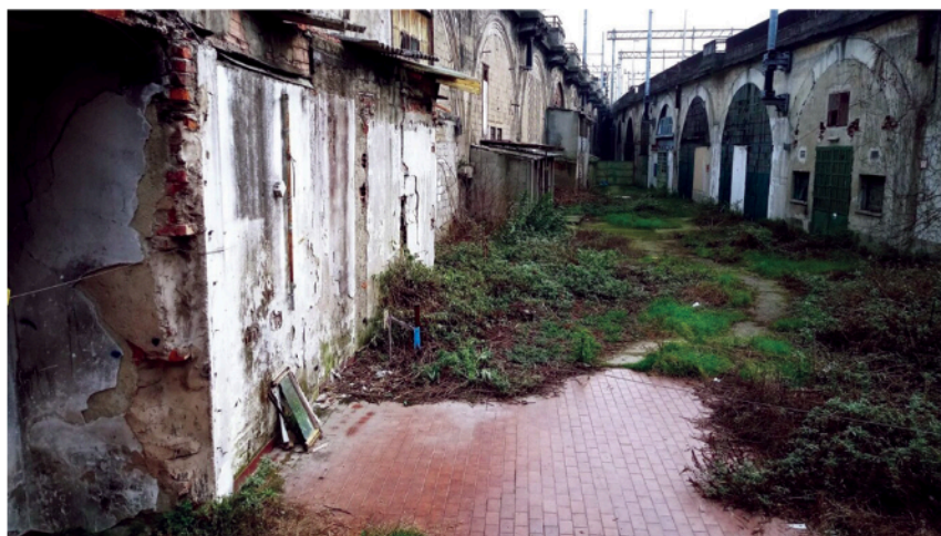
Fig. 2. The area prior to redevelopment. © ABCittà.
