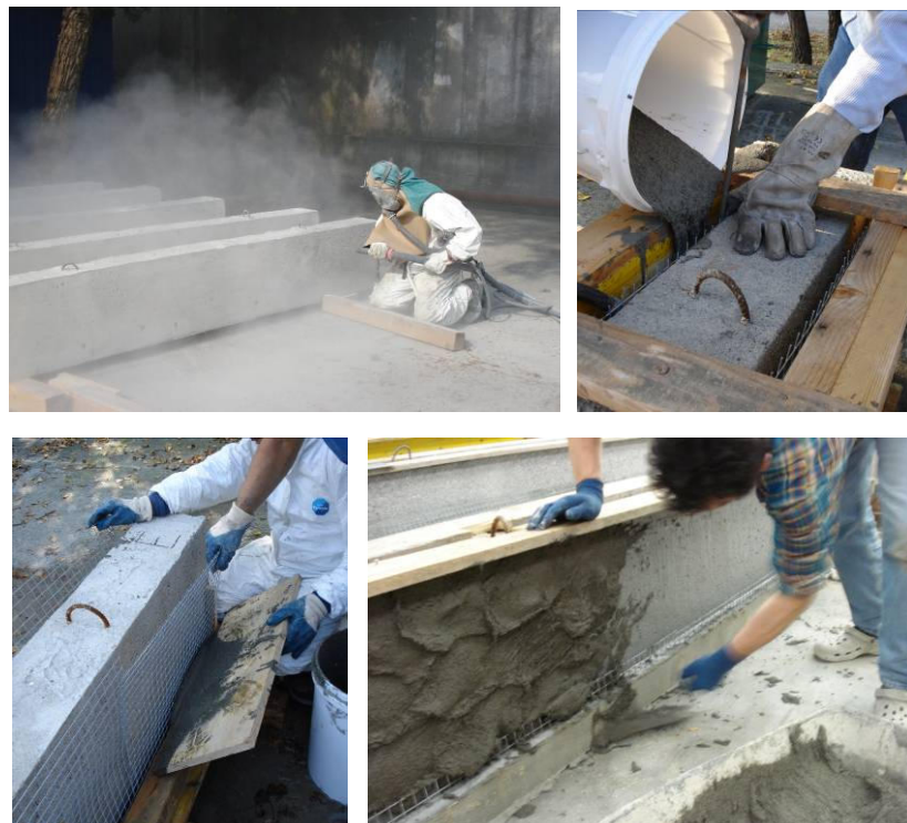
Fig. 1 Sandblasted and jacketing application.
