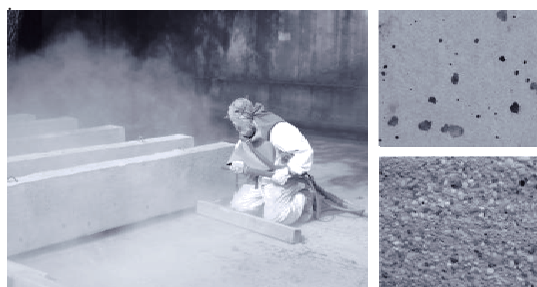
Figure 3. Sandblasting (left-hand); and surfaces before and after sandblasting (right-hand).
