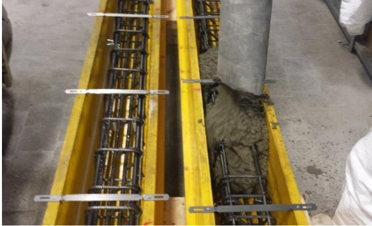
Figure 2.6: Concrete casting inside the formwork.
