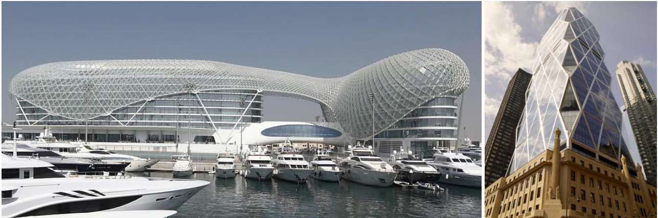
Figure 4 – Examples of a gridshell structure: Yas Viceroy Abu Dhabi Hotel ©Asymptote Architecture (left); and a diagrid structure (a particular type of gridshell): Hearst Tower, New York ©Foster+Partners (right)
