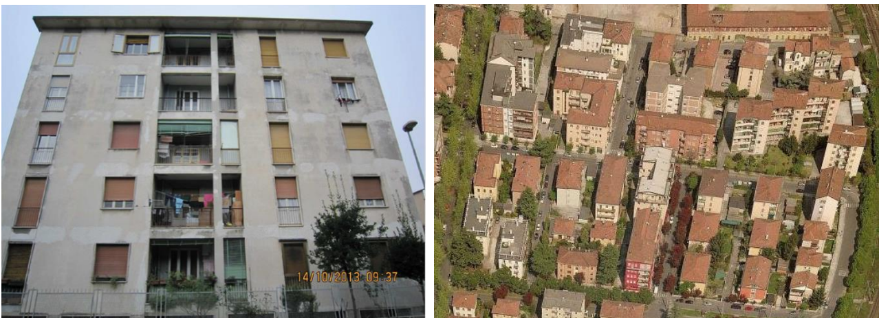
Figure 1 – Typical post-WWII European Reinforced Concrete buildings: a five-storey building with architectural, energy, and structural deficiencies (left) and a typical suburb (panoramic view © Microsoft® Bing™ Maps Platform 2016)
