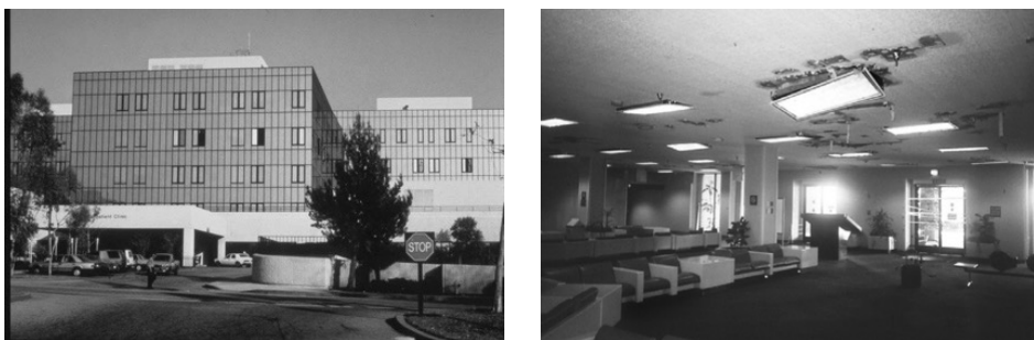
Figure 1.2 Olive View Hospital immediately after the Northridge earthquake in 1994 (left) and damage of the non-structural elements (right).
