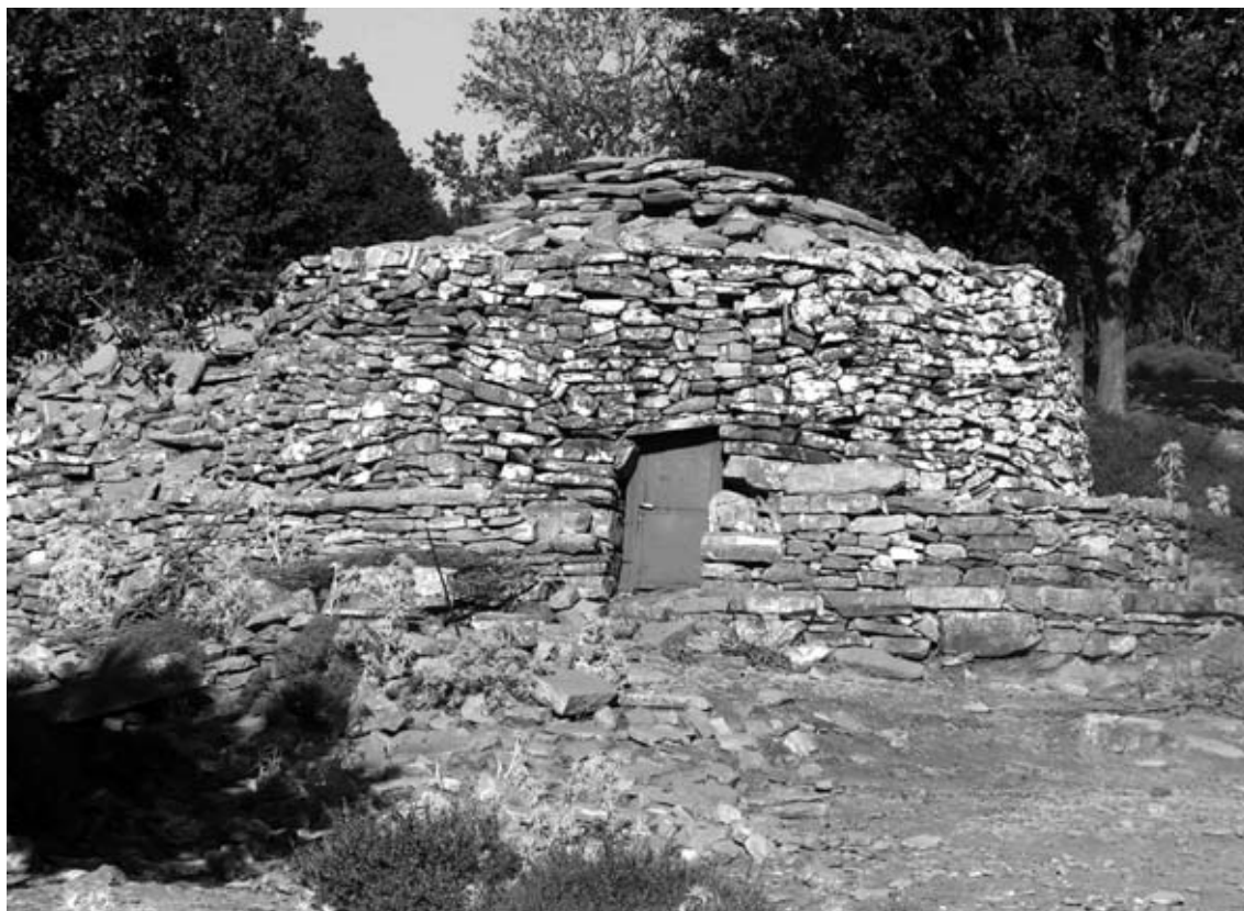
FIG. 3 – MITATO IN ZOMINTHOS AREA WITH THE VIEW OF ITS ROOFING TECHNIQUE.
