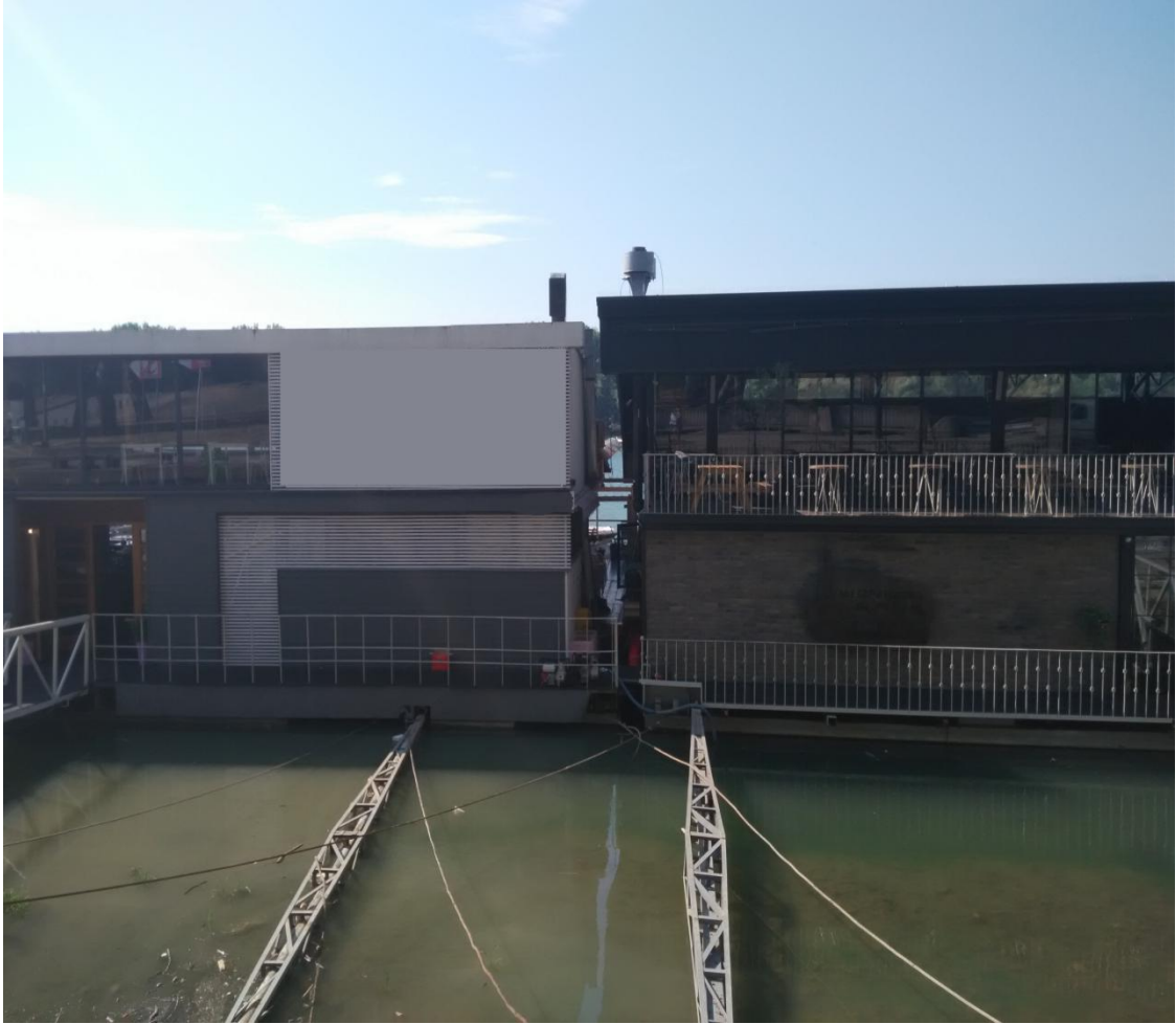
Image 6: Floating rafts are practically attached to each other with no space between them
