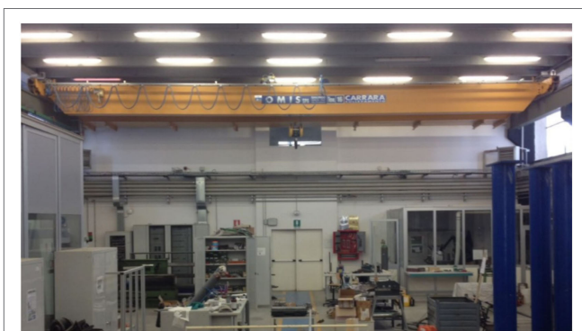
FIGURE 1 | Example of overhead crane in precast concrete buildings.
