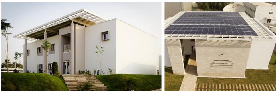
Fig. 2.1 - The Plus Energy building presented in November 2016
