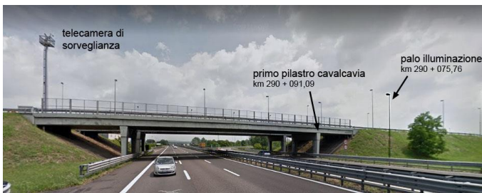
Figure 2. Lateral view of the bridge / Vista laterale del cavalcavia.
