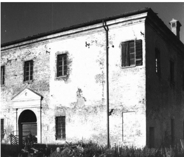
Figure 13: The main front of the villa in the 1960's. The crack due to the outward thrust exerted by the roof can be seen in the upper right corner (Private archive Alberto Ferrari).
