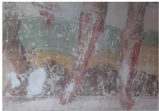
Figure 15: Wall paintings decay, room 4.
