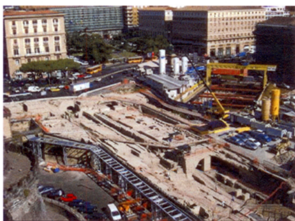
Figure 1. Overview of the site, july 2006
