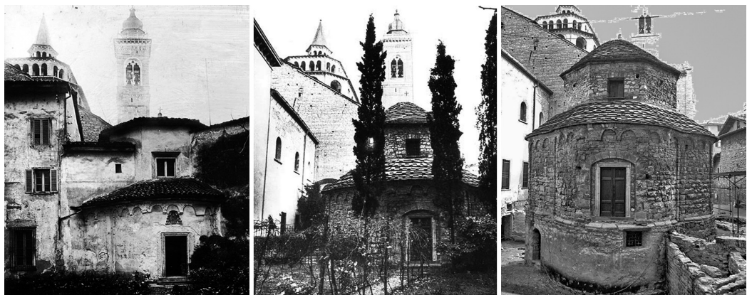
Fig. 6. The church of Santa Croce, before and after Luigi Angelini's restorations, and today.
