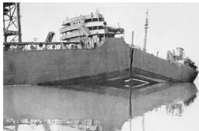
Figure 1: a) jet airplane Comet fuselage fatigue damage and b) liberty ships complete fracture [1-7].
