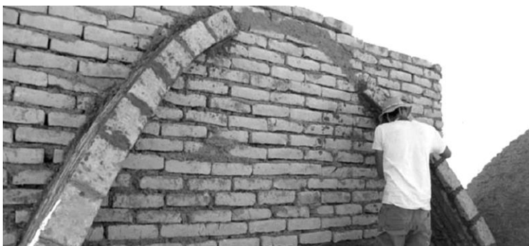
Figure 2.1.2 Pitched vault under construction. Photography by Adobe alliance [16].
