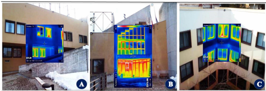
Figure 88: Outdoor thermography: (a) walls with north-west exposure; (c) inner courtyard wall.
