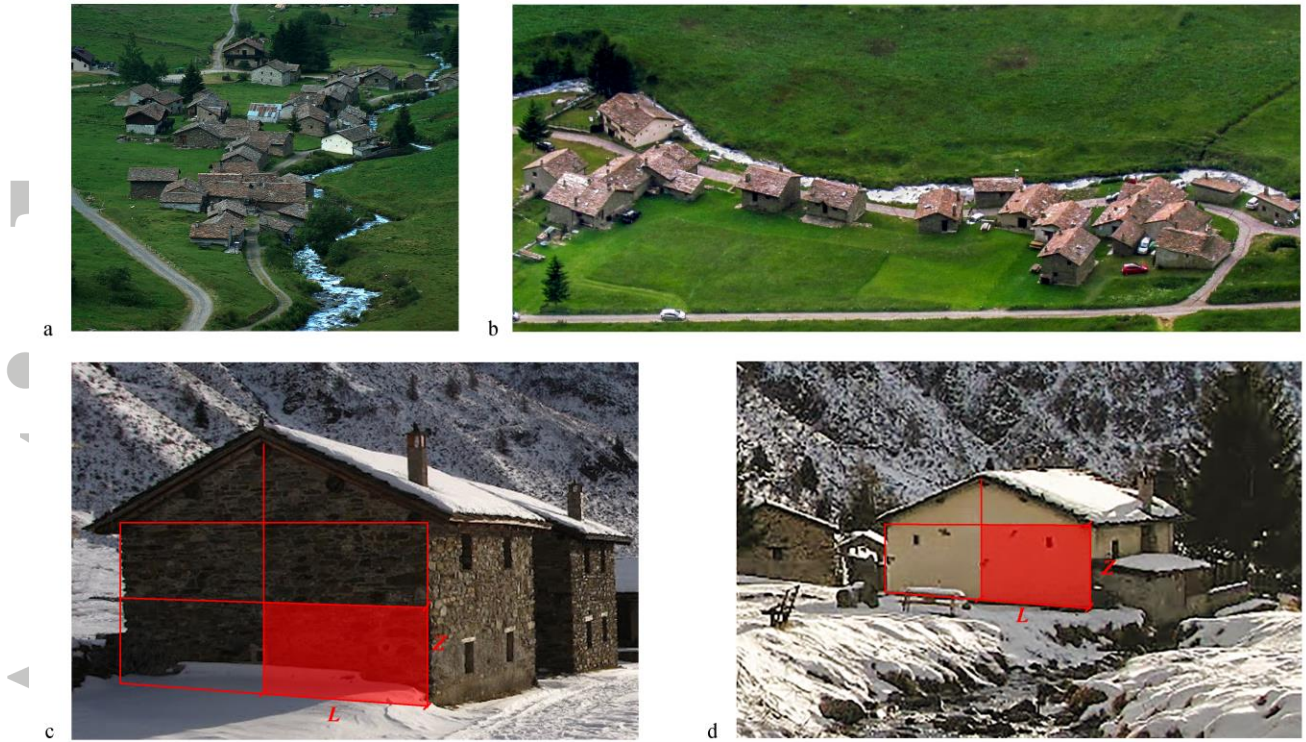
Fig. 1 – A traditional alpine village with a large stock of exposed masonry buildings in the Province of Brescia (Northern Italy) (a, b) and two examples of masonry buildings with indication of the most exposed walls (c, d).
