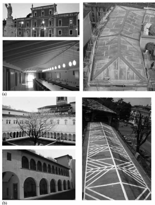
Figure 1: Examples of folded roof diaphragms adopted for the retrofit against vertical loads of some monumental buildings in Brescia, Italy: (a) University head quarter (exterior perspective view of the building, internal view of the existing wooden joists and top view of the strengthening plywood folded roof diaphragms with edge steel plate chords, overlaying the existing wooden roof, 2001); (b) Head administrative office of the University hosted in the former San Faustino Monastery XV century (exterior perspective views of the building, and top view of the plywood folded roof diaphragms further strengthened with additional strengthening steel stays, 1990; (Giuriani 1997).
