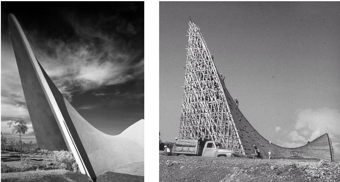
Figure 3. The Cuernavaca chapel finished and under construction.
