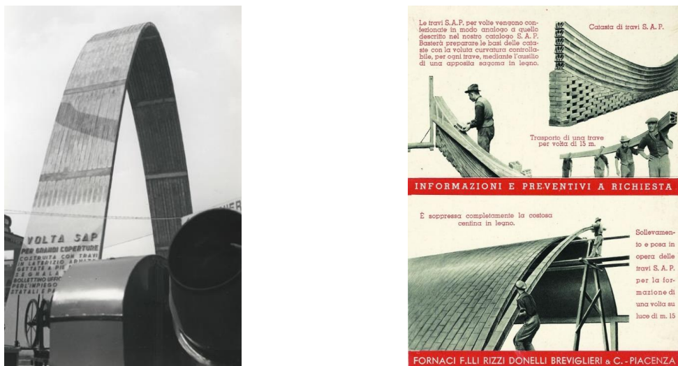
Figure 5. The vault built at Milan Fair in 1938 and a leaflet of SAP vault system.
