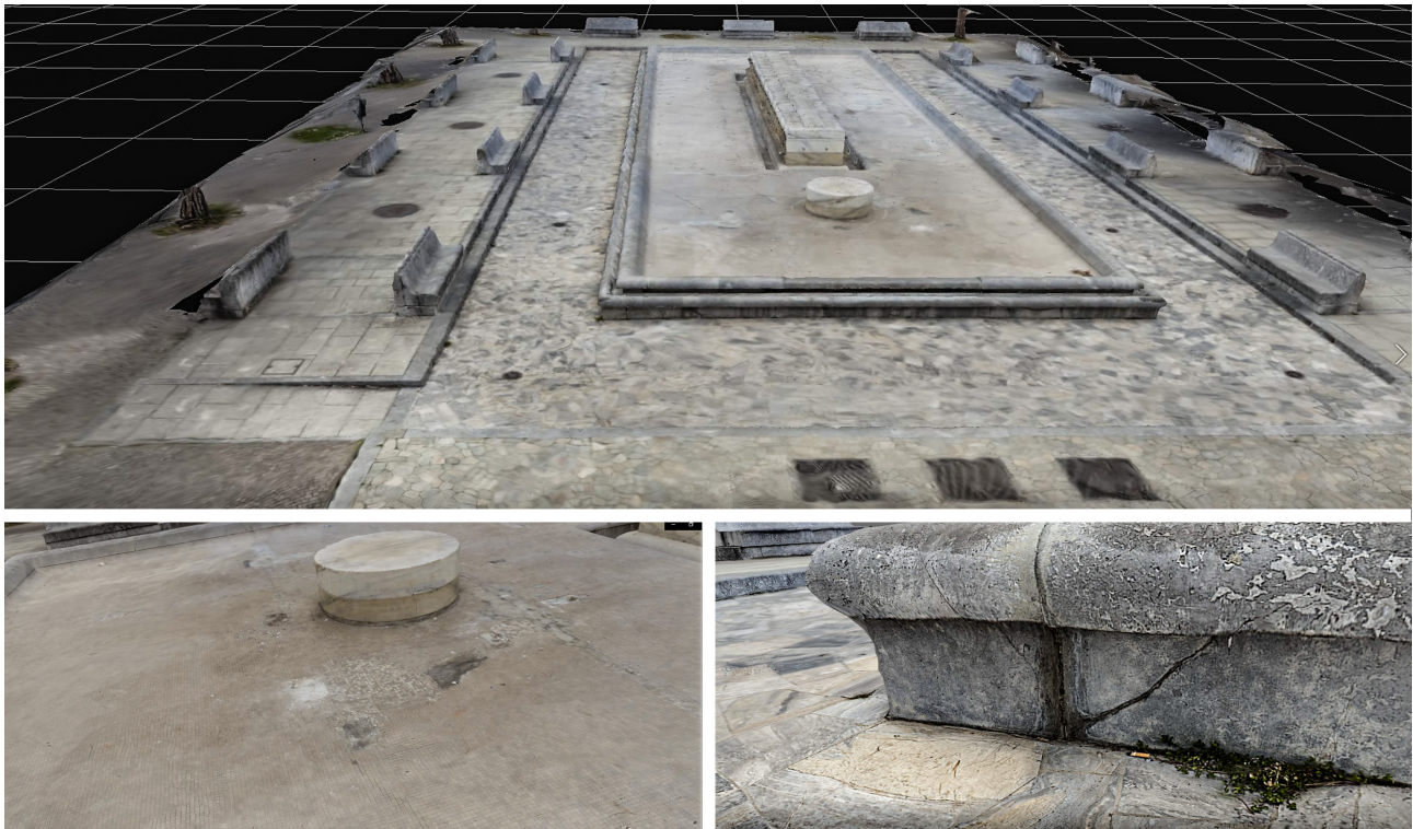
Figure 8. The Digital Photogrammetric survey: details of the textured mesh model
