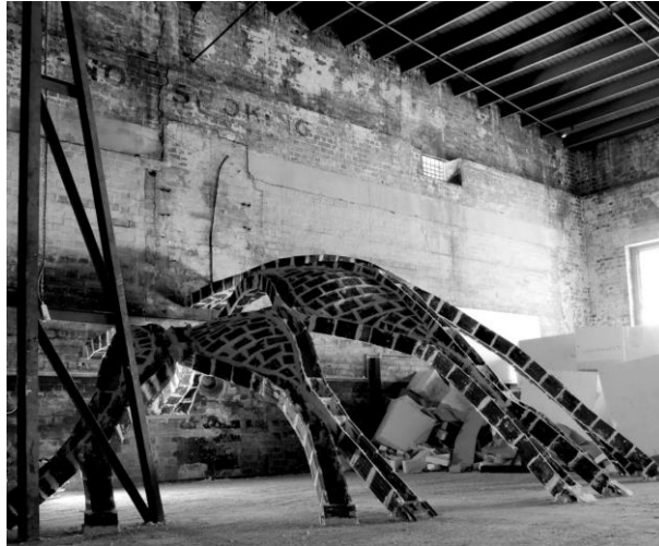
Figure 8: Complex ribbed vaults. Masterclass - Ribbed Catalan. Photography by M. Ford [52]
