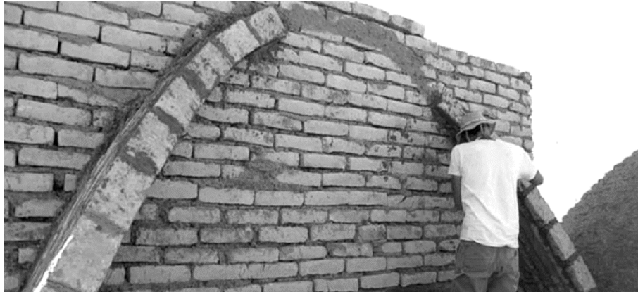
Figure 2: Pitched vault under construction. Photography by Adobe alliance.
