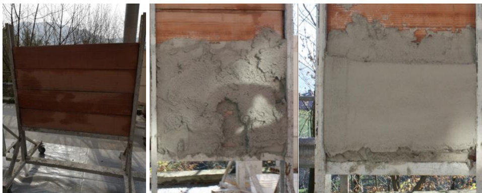
Figure 4-2 Application test: Support (left), application of plaster S8 4:1 MEF (middle) and application of plaster S8 4:1_def
