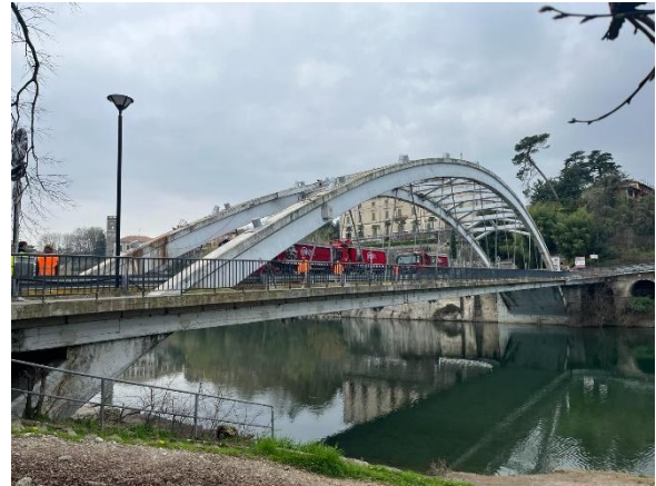
Figure 180: Load scheme used in the static load test and photo of trucks during the test.
