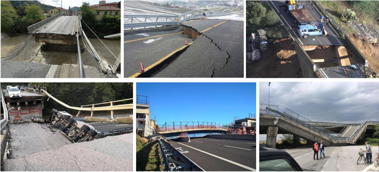
Figure 60: Example of collapsed bridges.
