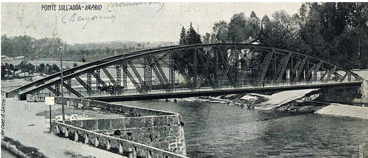
Figure 90: Historical photo of the old steel bridge.
