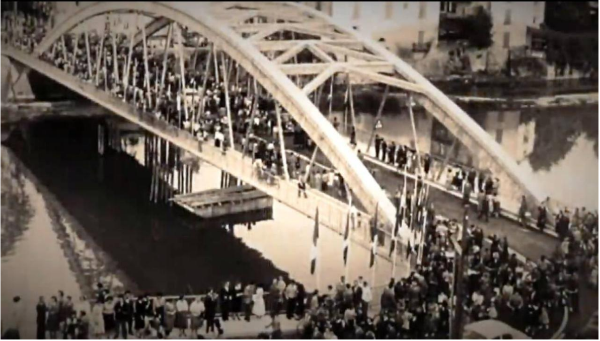
Figure 89: Historical photo of the Canonica bridge.
