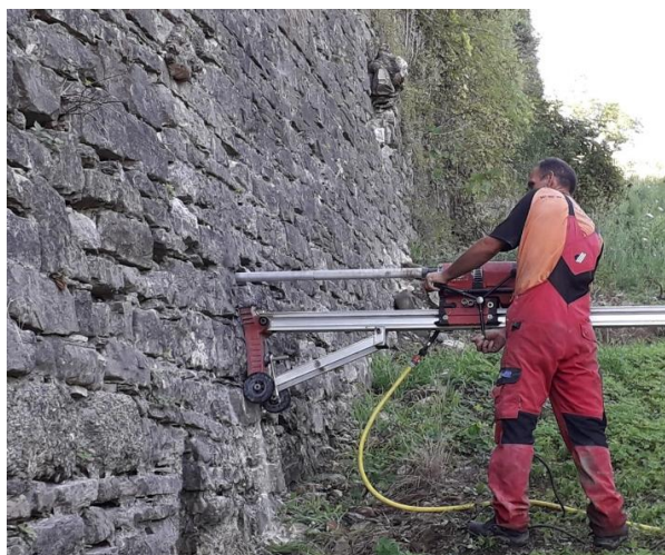
Fig. 2. Core drilling in the masonry carried out by Ecogeo srl.
