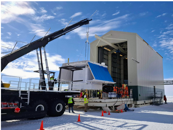
(a) Crane operations moving the fully assembled GAPS payload from the high bay at the LDB facility to the launch site.
