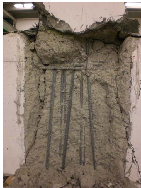
Figure 13. The joint after HPFRC jacket removal.
